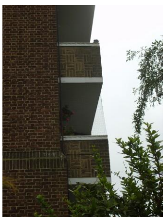
An example of netting used to protect a balcony.
